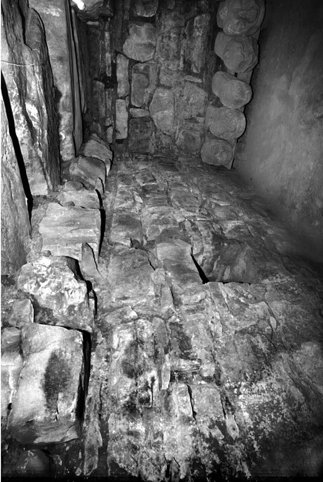
Figure 2.7. Chavín de Huántar's internal architecture: a room in the Laberintos Gallery. Note the pegs integrated within the ménsula course. The tenon heads were temporarily placed in this room for storage. Photo: Carlos Rodríguez.
