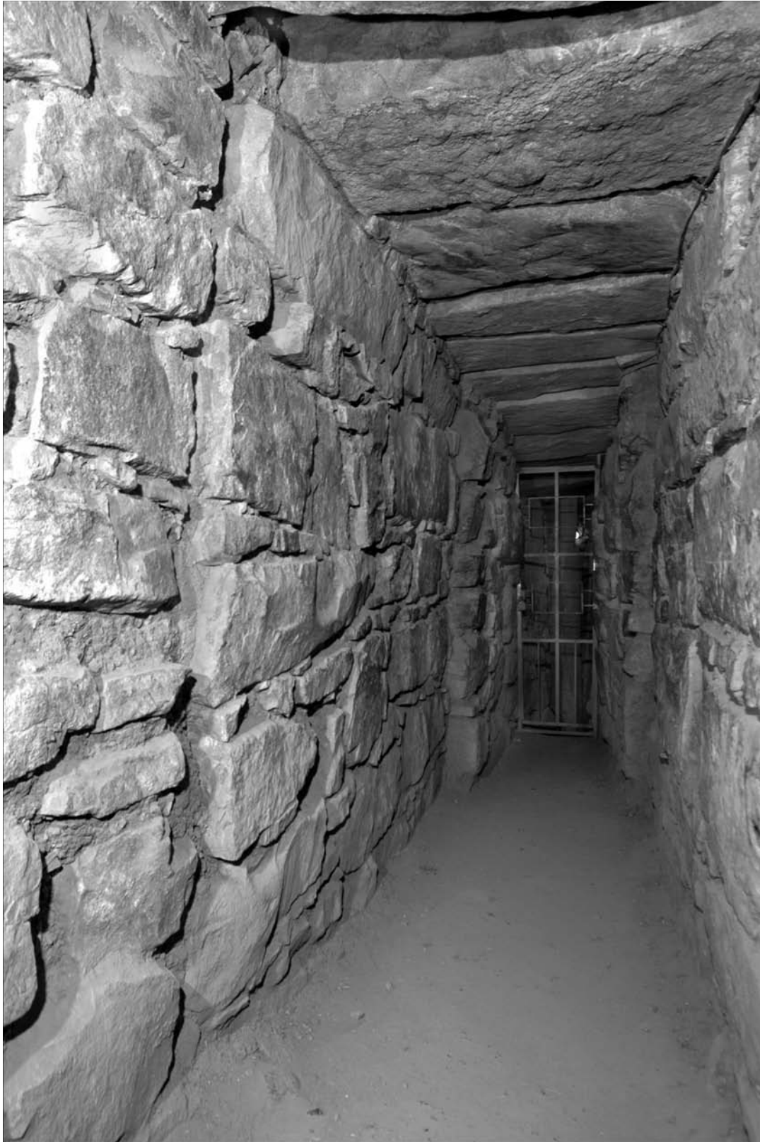
Figure 2.4. Chavín de Huántar's internal architecture: in the Lanzón Gallery, a hallway with construction seams. Seam Lan-E-3 is visible in the foreground; Seam Lan-E-2 is visible in the midground; Seam Lan-E-1 is at the gate. The Lanzón monolith is behind the gate. Photo: John Kembel.
