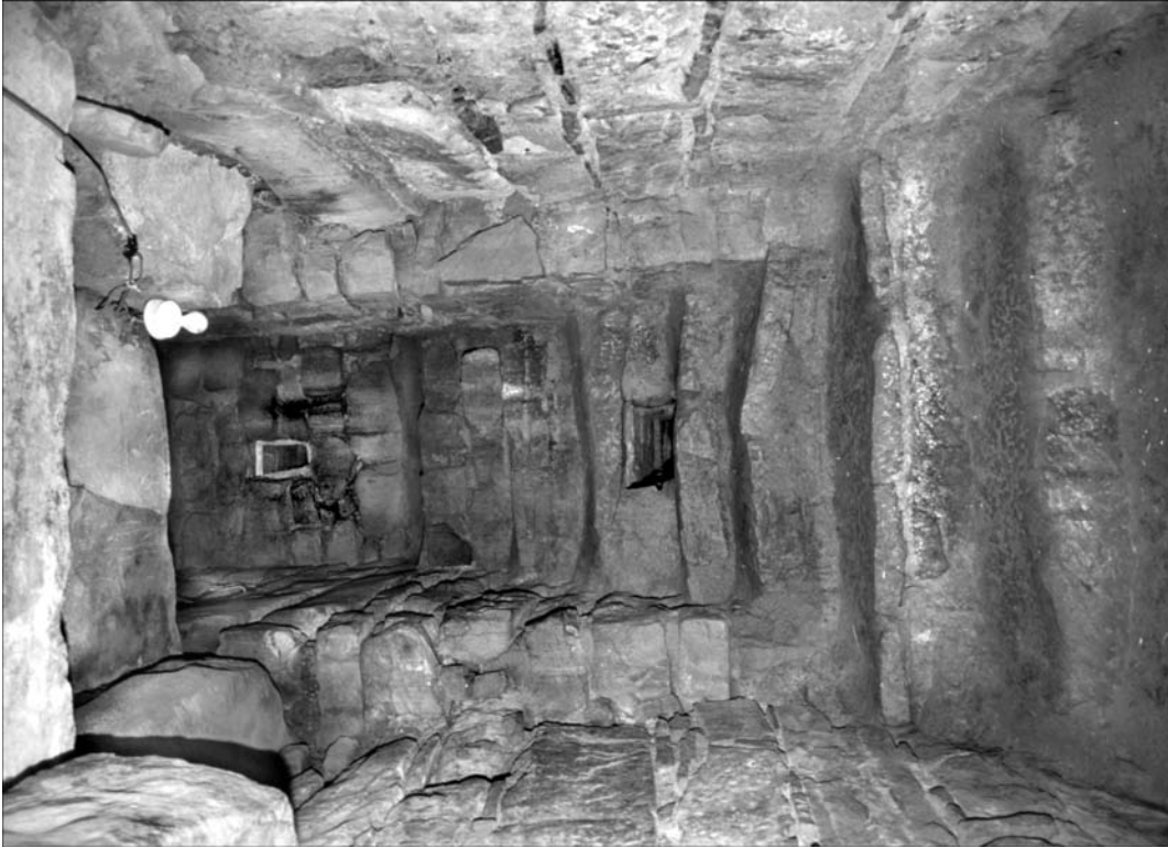
Figure 2.6. Chavín de Huántar's internal architecture: staircase with- in the Doble Ménsula Gallery, with two ventilation shafts. A construc- tion seam is present between the staircase and the end of the hallway. Photo: Carlos Rodríguez.
