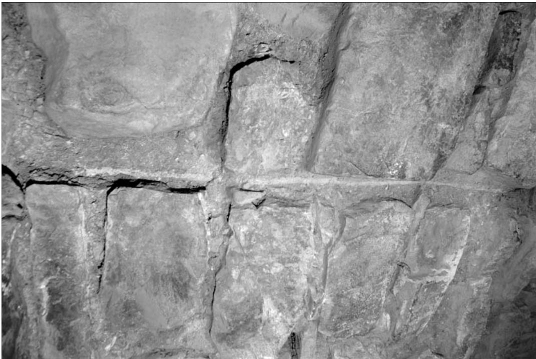
Figure 2.5. In the Lanzón Gallery, detail of Seam Lan-E-3, showing white plaster that marks the formerly exterior wall sur- face of the Lanzón Patio. Photo: John Kembel.
