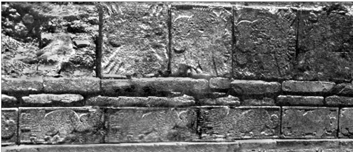
Figure 11.5. Interior wall of the circular sunken courtyard
