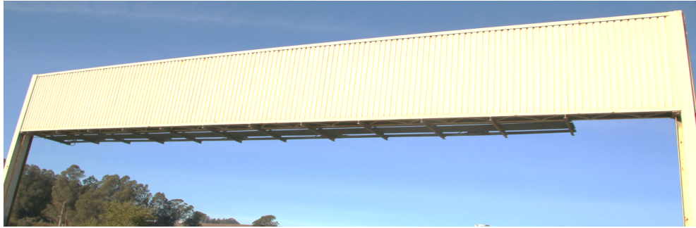
(a) Photograph of the overhead sign structure.
