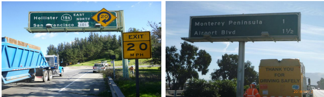
(a) Single post cantilever structure, Location 24, OSMI ID: 44156005239EB1 (b) Single post butterfly structure, Location 20, OSMI ID: 44101087286SB1
