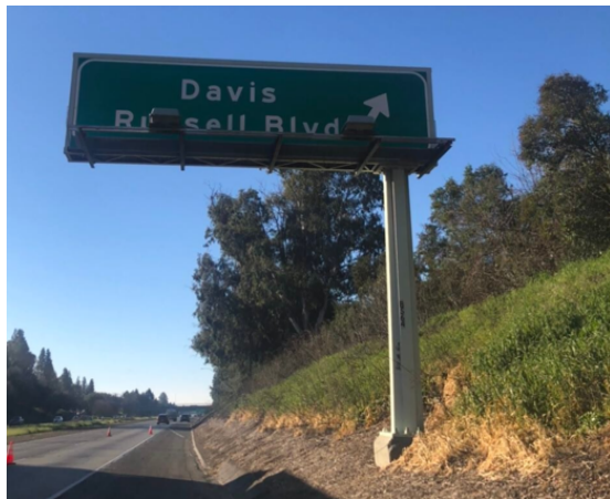
(a) Photograph of the sign structure
