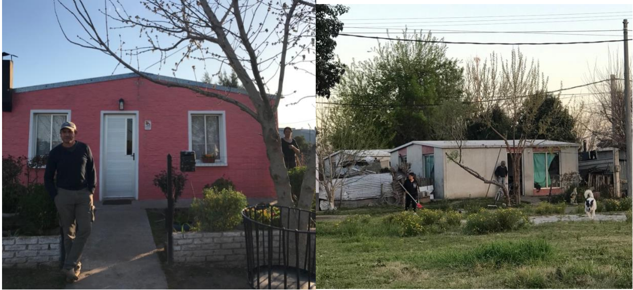
Figure 33: To the left is a MEVIR home built after the 2016 tornado in Dolores, Soriano Department. To the right is a nearby home built after the same disaster by a company called Schmidt (photo by author, 6 September 2022).
