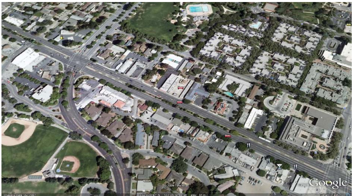
Figure 2.1.b. Median space unused or underused for traffic purposes: The section of the W. El Camino Real in Mountain View, California, USA between S. Shoreline Blvd. and Castro Street, shown as the street oriented diagonally
