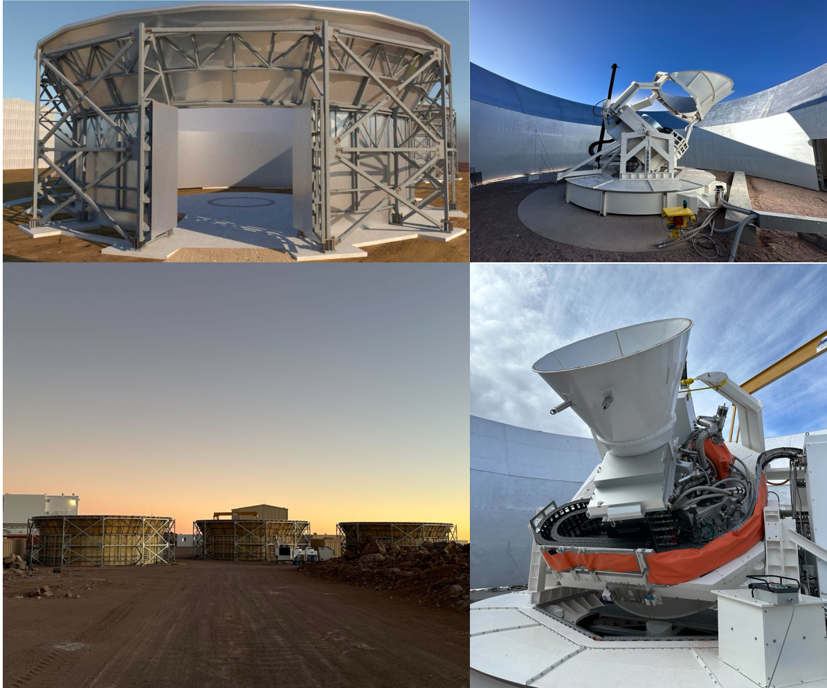
Figure 4.11. An overview of the ground shield and other warm baffling. Top Left: A solidworks model of the ground shield. Top Right: The interior of the ground shield, with the co-moving shield mounted on the SATP. Bottom Left: All three ground shields fully constructed on site. Bottom Right: The interior of the ground shield with the SAT receiver forebaffle, but no co-moving shield. Pictures taken by Michael Randall, model by Grant Teply.
