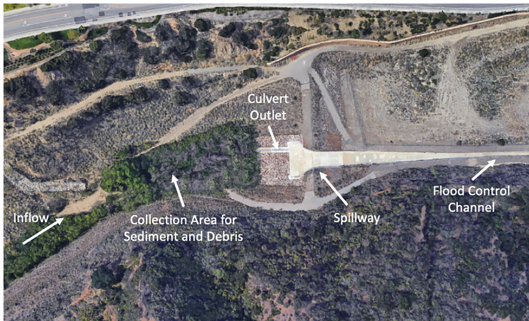
FIGURE 2 McVicker debris basin in Riverside County, California. Coarse sediment and debris settle in the collection area, while flood water and suspended fines pass through a culvert into a flood control channel. A spillway is used to accommodate high flows. Image source: Google, 2018
