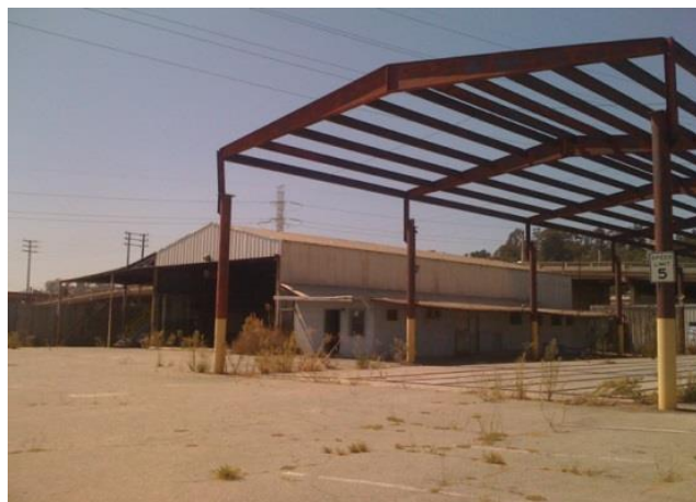
Figure 6. Albion Riverside Park Project Picture Showing Before Construction (Source: LA Sanitation & Environment).
