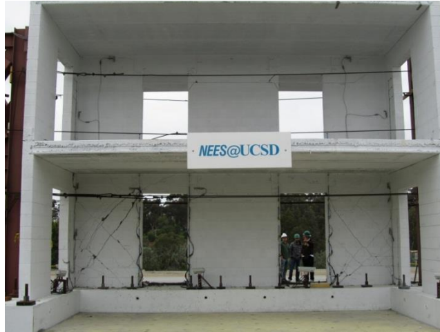
(a) Shear failure of reinforced masonry walls
