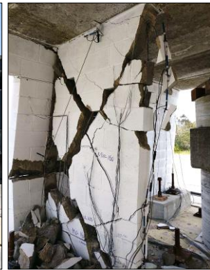
(c) South view of Wall-1
