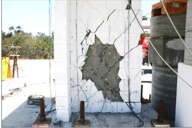
(a) South view of Wall-1
