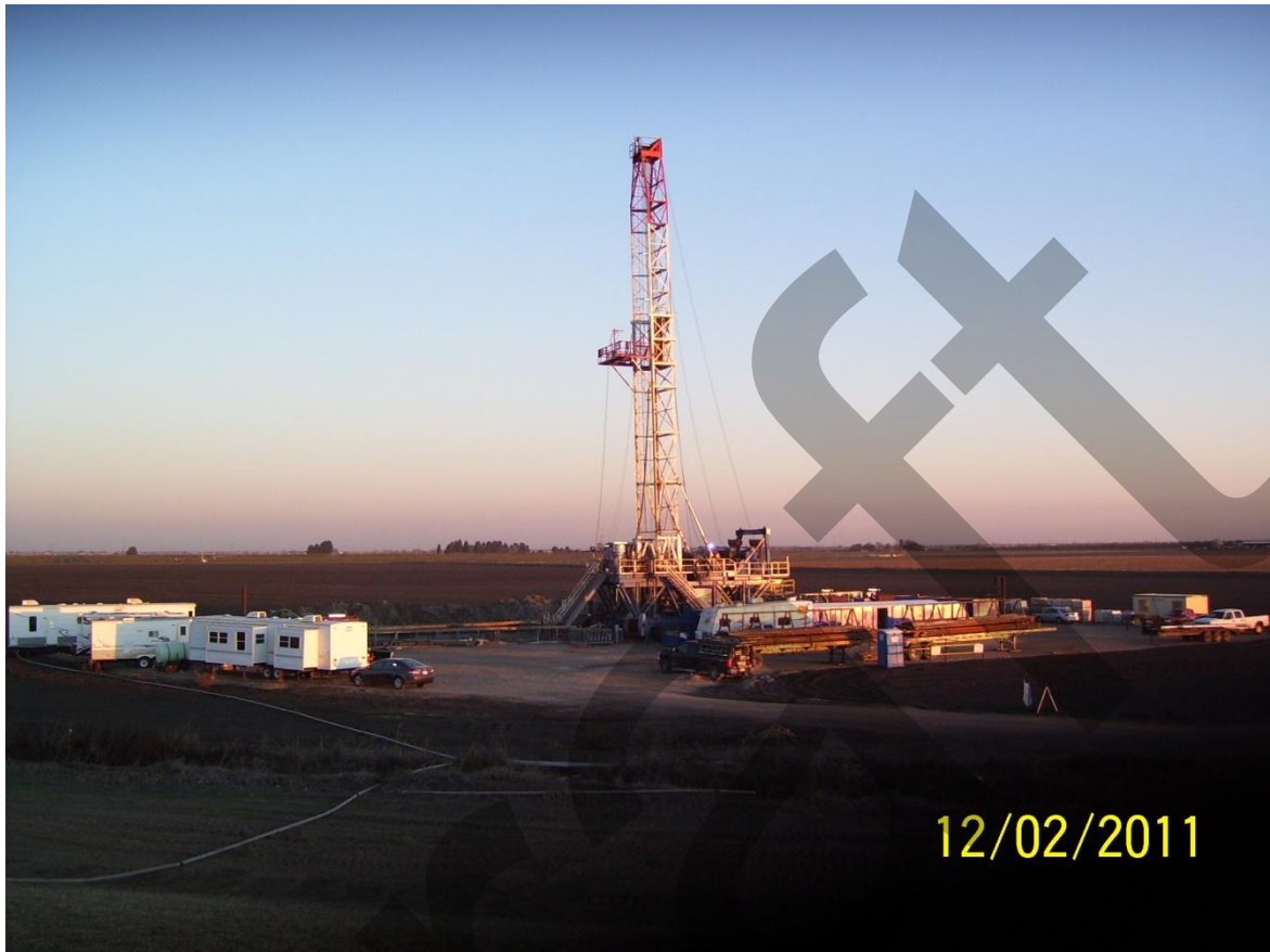
Figure 10. Citizen Green Well 1 drill rig at King Island.
