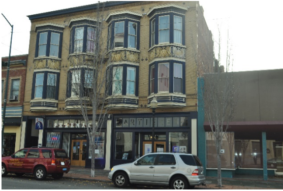
Example of Vallejo's Historic Architecture
