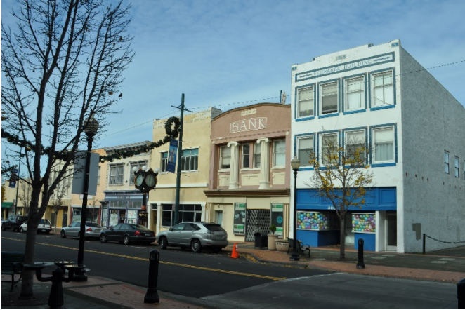
Example of Vallejo's Historic Architecture
