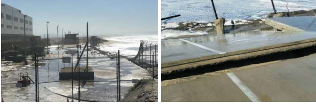
Figure 4.2: Photos of Coronado berm failure during March 5-7th, 2016 resulting in backshore parking lot flooding and undermining.
