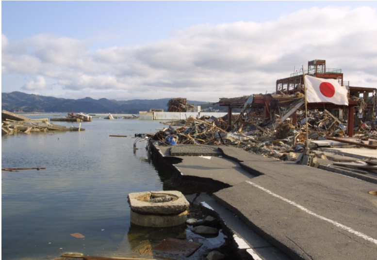
Photo 4.1: Hinomaru in Minami-Sanriku, Miyagi prefecture. Source: BLOGOS 243
