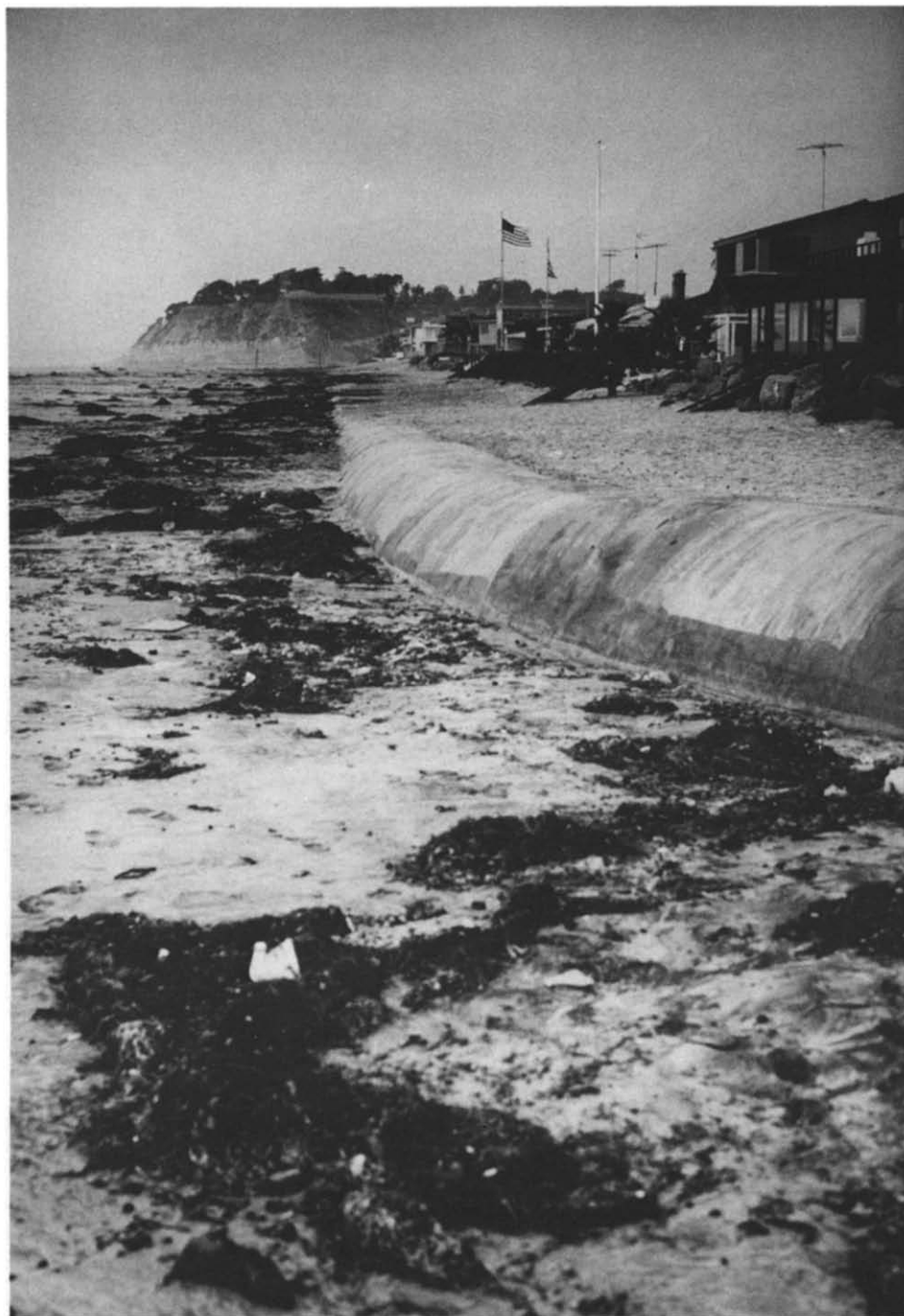
Fig. 8. Mild winter of 1981—1982 produced only minor removal of sand near Longard Tube. Photo 12 November 1981.
