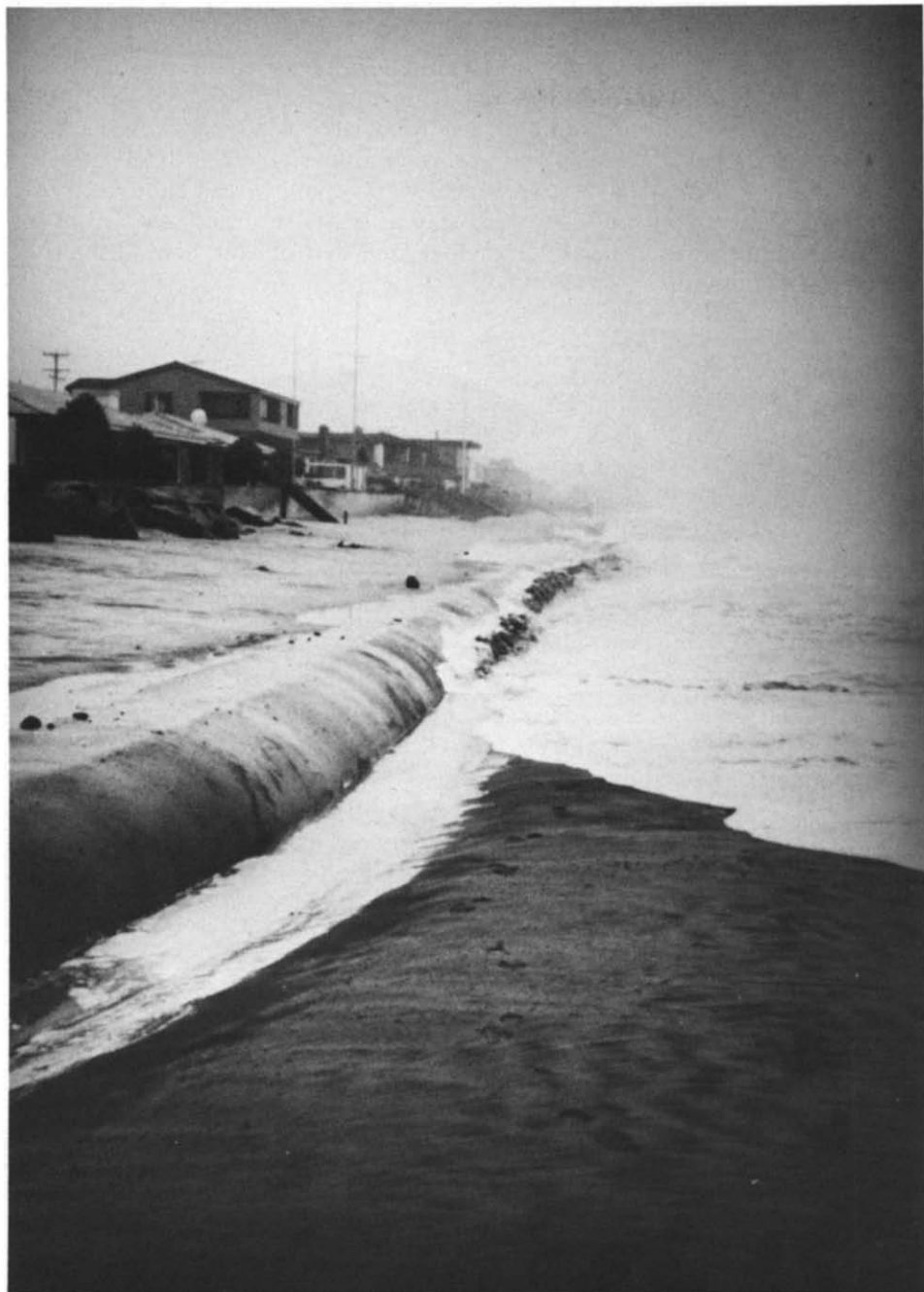
Fig. 2. Wave interaction with Longard Tube during first winter storm, 22 January 1981.
