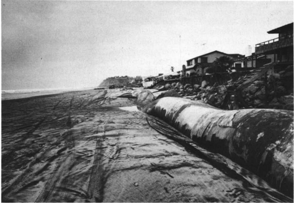
Fig. 14. Photo taken 28 January 1983 at low tide looking north and showing major undulations and scour depressions in Longard Tube. Note exposed filter cloth previously attached to 25 cm diameter toe protection tube now flung over stair case on shoreward side. Extensive rock rip-rap was placed all along Del Mar beach during the storm episode.
