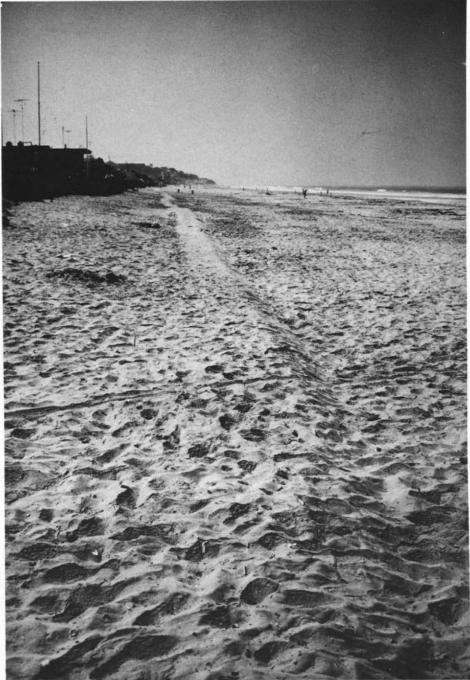
Fig. 6. Accretion of beach during late spring and summer 1981 essentially buried the Longard Tube and removed it from wave interaction. Photo looking south along tube axis taken 2 September 1981. See Fig. 6 for accretionary profile sequence.
