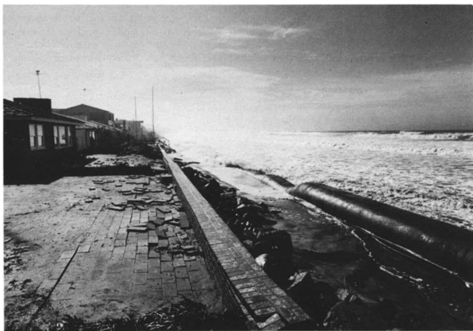
Fig. 13. Photo taken 28 January 1983 during 2–3 m high tide showing tube subsidence and undulations. Overtopping waves scoured sand from shoreward side of tube. Loose bricks on this patio and other property damage indicated maximum uprush of about 4 m above mean sea level.
