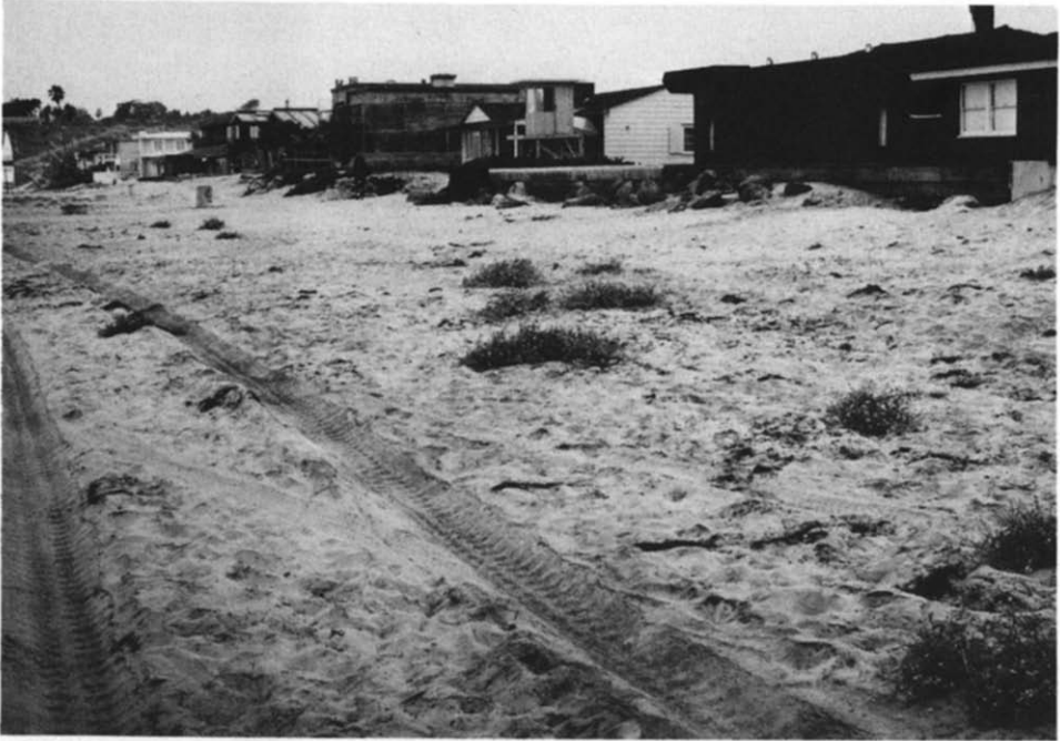
Fig. 9. Mild winter of 1981—1982 and continuing accretion caused Longard Tube to be completely buried by date of this photo (looking north) 28 June 1982.
