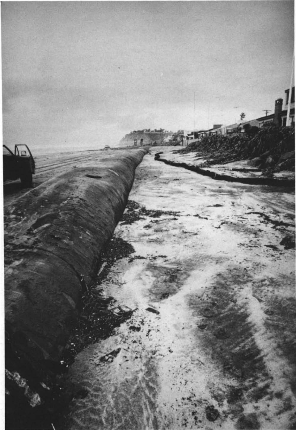
Fig. 12. Photo taken 27 January 1983 showing severe beach erosion, particularly sand removed from shoreward side of Longard Tube. Note 25-cm tube intended as toe protection for main tube thrown shoreward.
