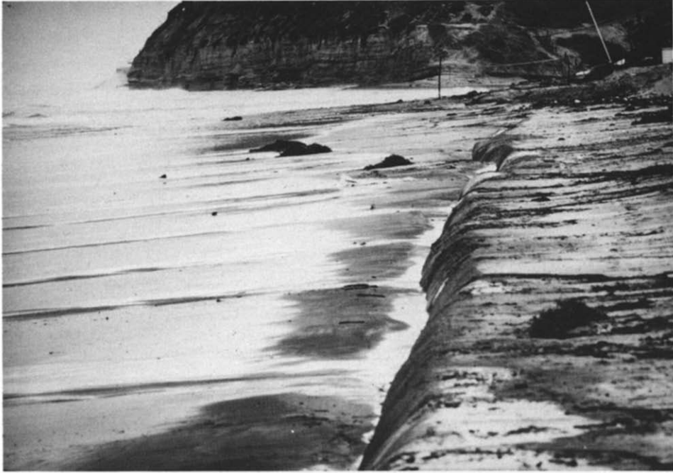
Fig. 4. Photo taken 5 March 1981 showing first stages of localized scour depressions on the seaward side of the tube formed by seaward return flow over tube at points of lowest vertical elevation. This photo taken after the tide had dropped and shows only the remnants of the scour channels which are filled in as over-topping of the tube ceases.
