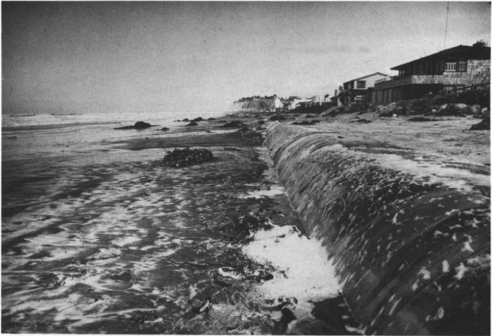
Fig. 10. Photo taken 2 December 1982 showing perched beach and substantial removal of sand seaward of Longard Tube during first winter storm of 1982—1983. Profile change and tube subsidence shown in Fig. 12.
