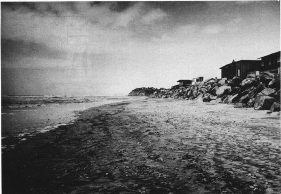
Fig. 17. Photo looking north from Range 2 (foot of 25th Street, see Fig. 15) on 24 March 1983 after removal of Longard Tube. Note rip-rap revetment and very low sand level due to extreme winter erosion.
