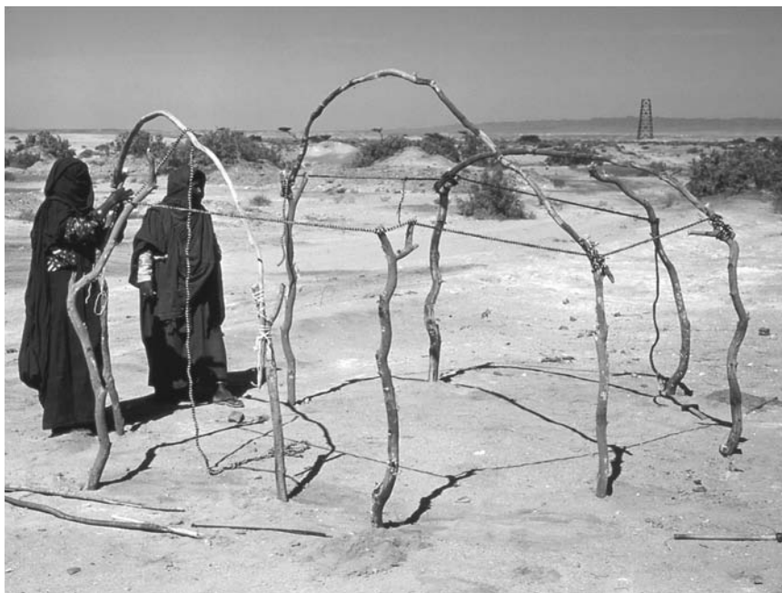
Figure 23.10. Building a beit al-burush : forked acacia branches and roots are secured into the ground and tied into a frame.
