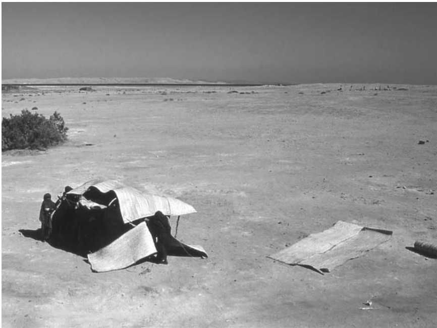
Figure 23.13. Building a beit al-burush : the outer walls of the house are made of large doam palm leaf mats.
