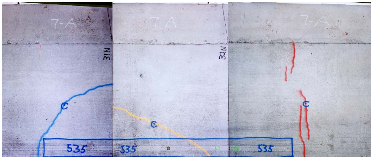
Figure 32. Composite image of Test 535FD showing cracks.
