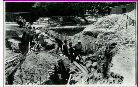
2) Excavation to install infrastructure began
