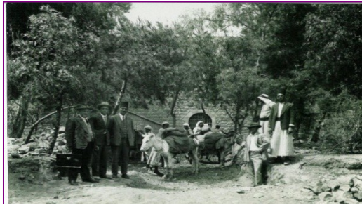
1) Engineers and workmen gathered at the construction site
