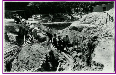
2) Excavation to install infrastructure began
