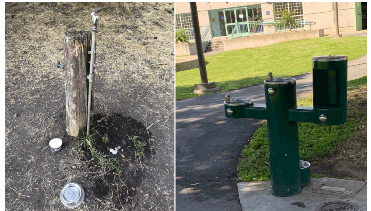
Figure. Drinking fountain in a comparison park (left) and Drink Tap water station in an intervention park (right). The Drink Tap water stations were installed in winter 2017.
