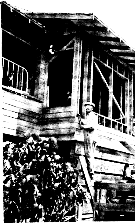
Dad nailing siding to Normal Street House
