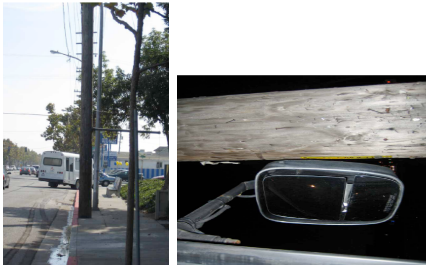
Figure 25 Utility Pole near Station #1 (right: 6" to curb; left: bus mirror next to pole when the bus is 20 cm to the curb)
