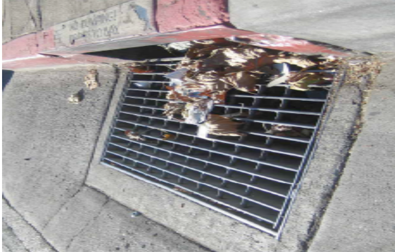
Figure 28 Storm Drain in front of Station #1
