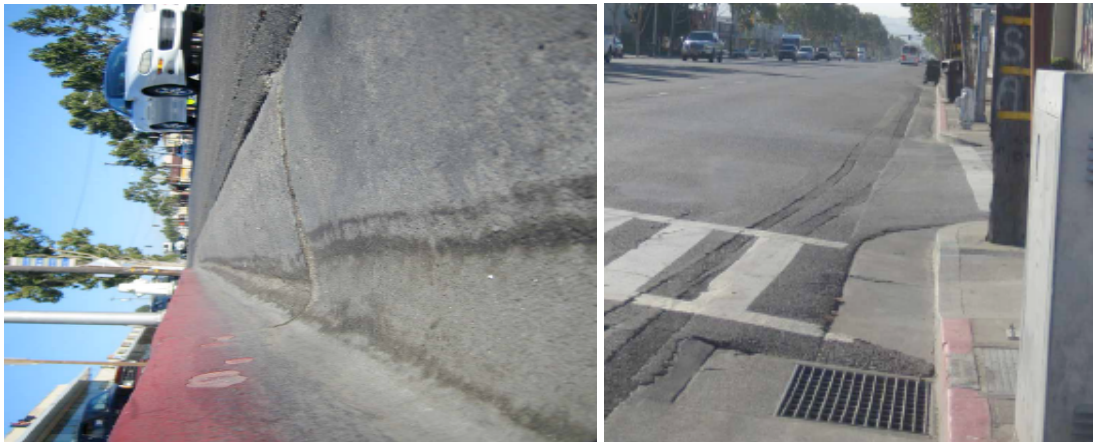
Figure 27 Road Crown before Station #2 (4.75-4.15 degree); Right figure: Notice Road Crown from the Crossroad – 144 Ave.
