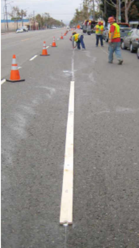
Figure 19 East 14 th Street Installation: Wooden 10m Template.
