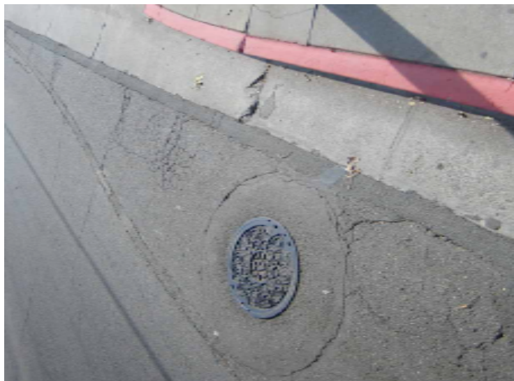
Figure 29 Utility access cover in front of Station #1
