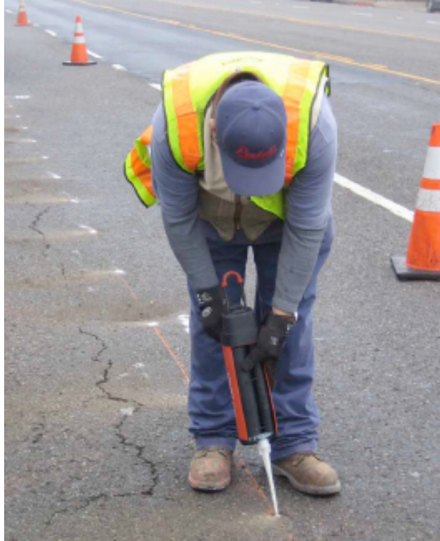
Figure 22 East 14 th Street. Installation: Sealing Magnets
