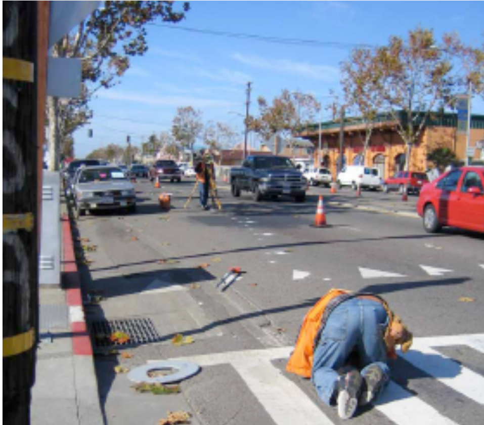
Figure 17 East 14 th Street Installation: Survey and Mark (1m around station, 10m otherwise) on the Ground
