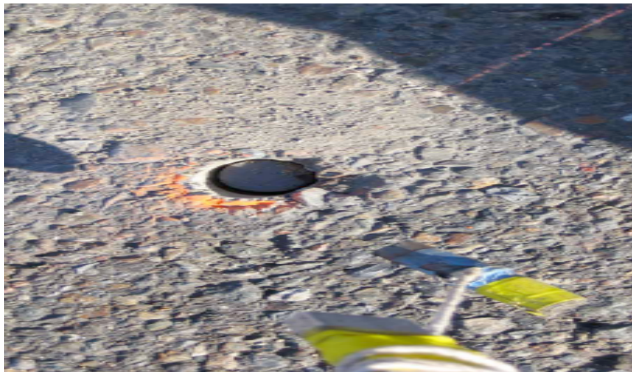
Figure 21 East 14 th Street. Installation: Placing Magnet and Checking Polarity (with home-made tool)
