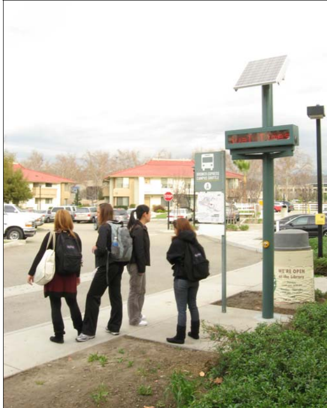
Figure 6 Solar-Powered Sign at the University Village Bus Stop
