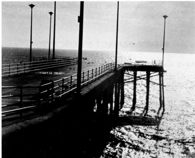
Figure 5. Abrupt end of Huntington Beach Pier photographed 20 January 1988. The seaward 250 feet of pier and "The End" Cafe were washed away Sunday evening 17 January 1988.
