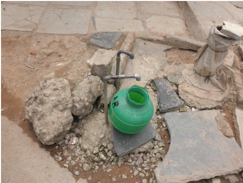
Figure 4. Public Water Taps in Indiramma Nagar, Rasoolpura
