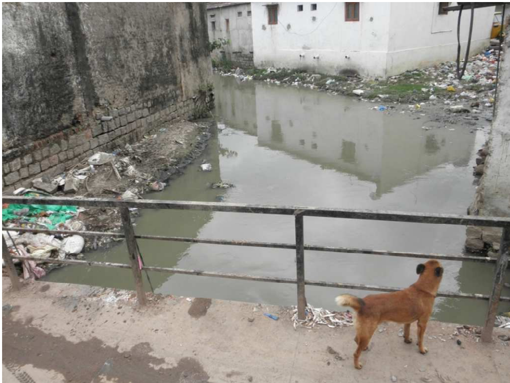
Figure 6. Open Drain Transecting Rasoolpura Settlement
