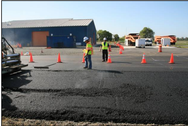
Figure 2.28: Control #1: Chunks in mix.
