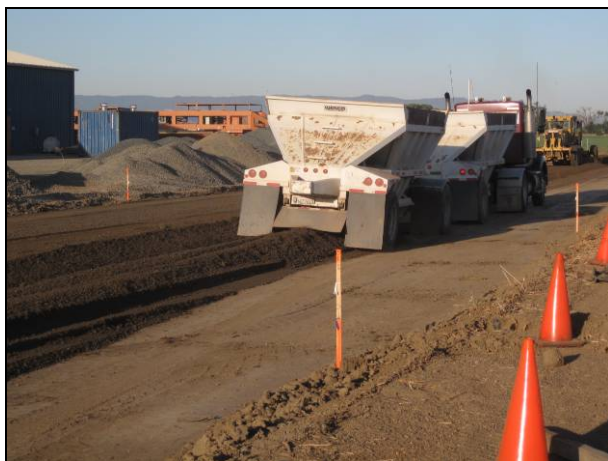
Figure 2.15: Dumping material in windrows.
