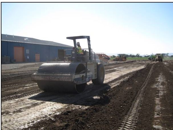
Figure 2.12: Final compaction.
