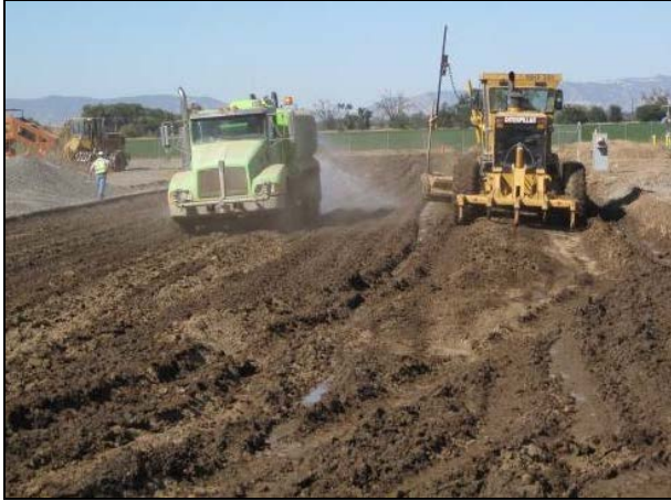
Figure 2.8: Watering and mixing.
