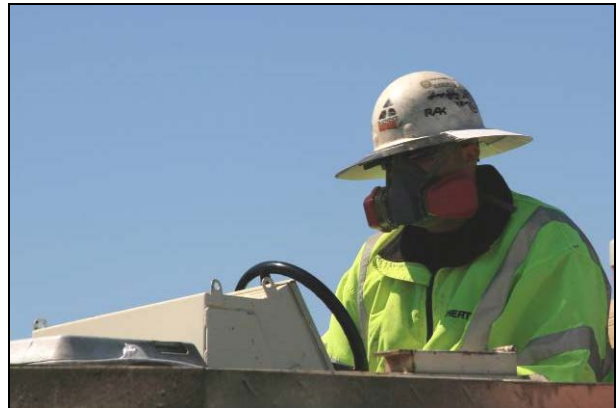
Figure 2.30: Control #1: Paver operator wearing respirator.
