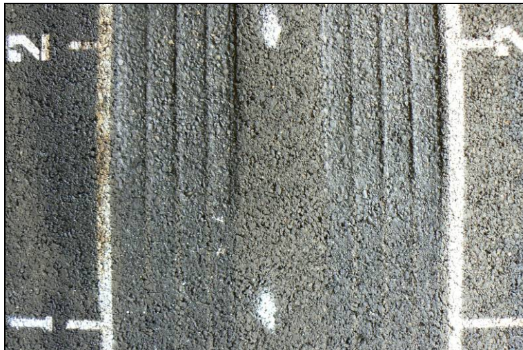
Figure 4.11: 624HB: Section photograph at test completion.
