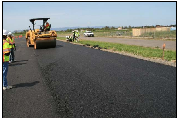
Figure 2.44: Rediset: Breakdown rolling.
