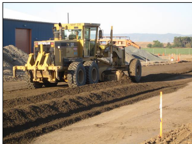
Figure 2.16: Material spreading.
