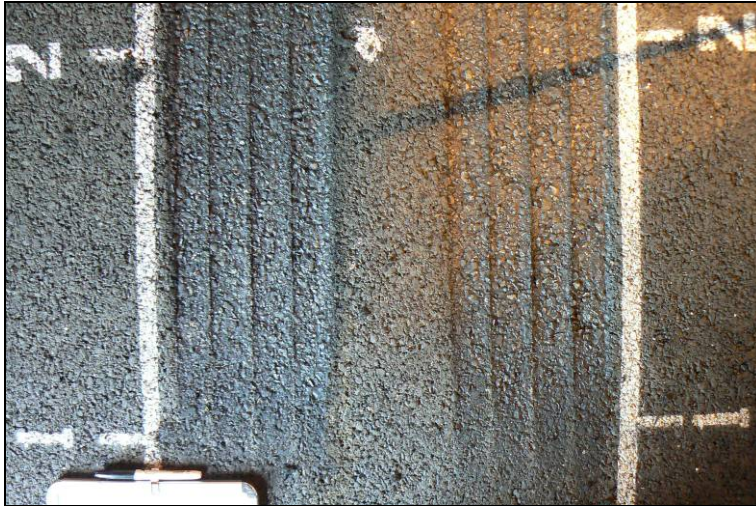
Figure 4.20: 625HA: Section photograph at test completion.
