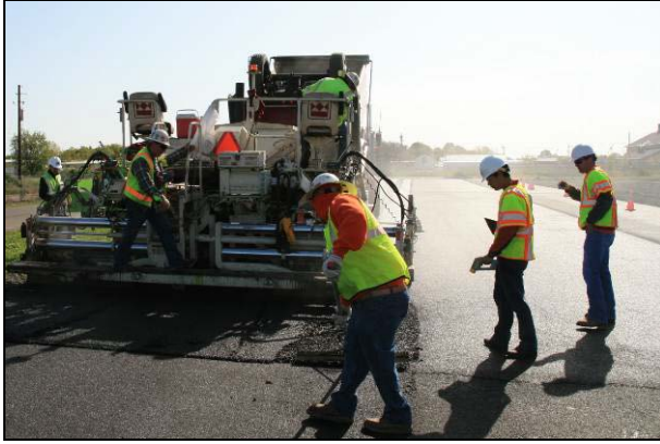
Figure 2.41: Astec: Some smoke from truck and paver.
