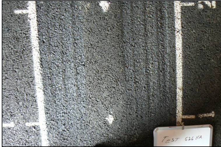
Figure 4.29: 626HA: Section photograph at test completion.
