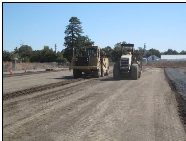
Figure 2.19: Heavy watering prior to pre-final compaction.
