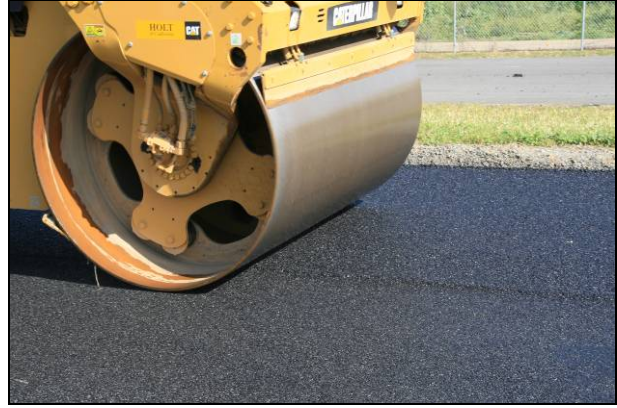
Figure 2.42: Astec: Breakdown rolling.
