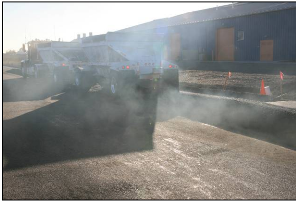
Placing asphalt in windrow
