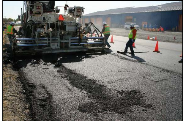
Figure 2.28: Control #1: Chunks in mix.
