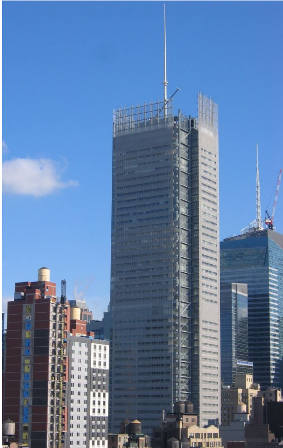
Figure 2.1.3-1: The New York Times Building, New York, NY
