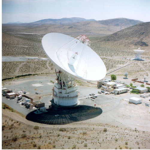
Figure 1.1: DSS-14 70 m reflector on an Alt/Az mount at Goldstone Complex [1]
