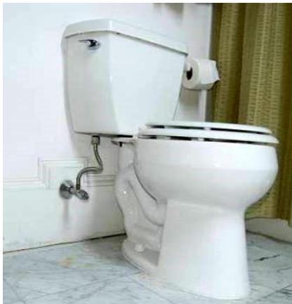
Flexible water supply connector, Flex Pipe, or Flexi Hose (Source: Picture by Iris D. Tommelein, Boston, MA, 2007)
