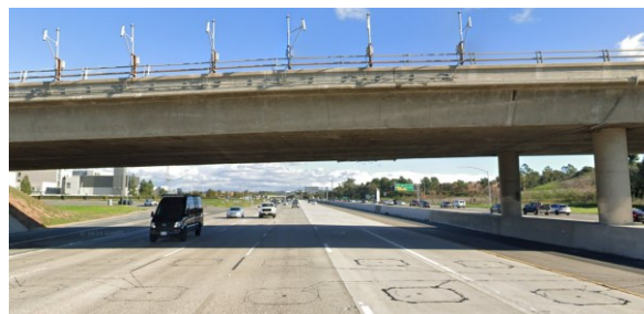
Figure 1.1. Inductive Loop Detectors and Video Cameras on I-405/Sand Canyon Drive
