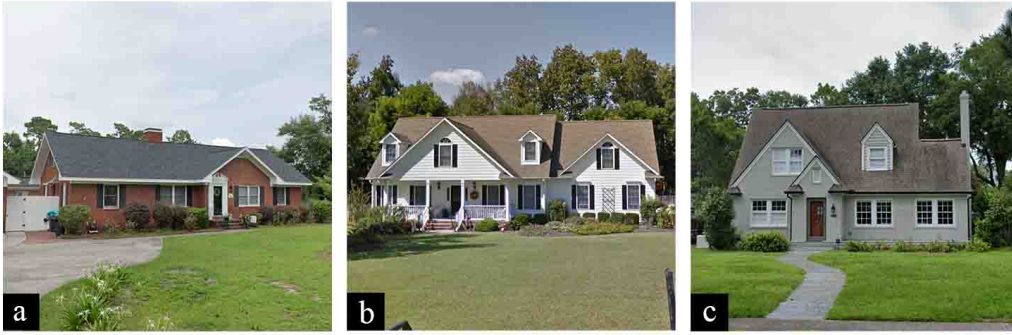
Figure 4.37: Representative single-family houses with attics and steep roofs. Roof pitch: (a) 8/12 ( 34^\circ ); (b) 10/12 ( 40^\circ ); (c) 16/12 ( 53^\circ )
