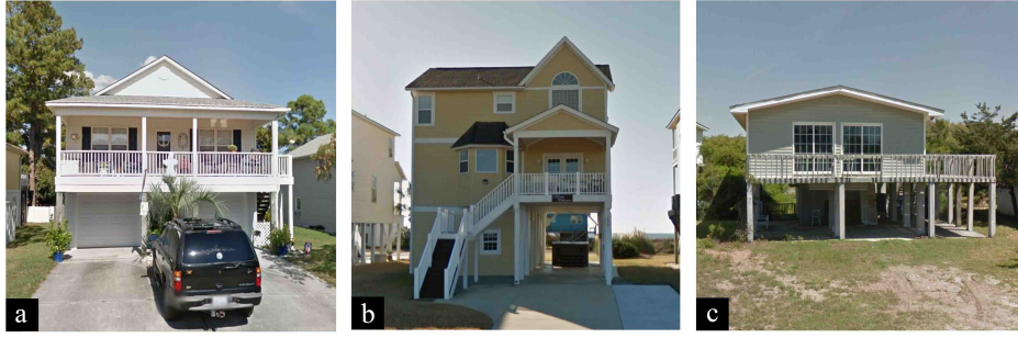
Figure 4.27: Typical elevated single-family houses with different enclosure condition of the base floor: (a) Enclosed; (b) Partially enclosed; (c) Partially open
