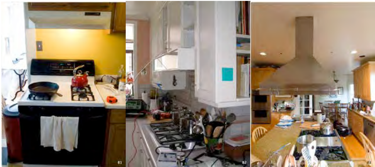
Figure 6. Exhaust systems with open capture hoods B1–B3
