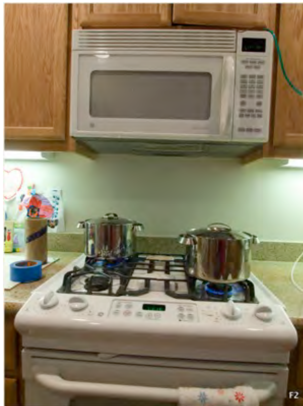
Figure 14. Microwave over range; exhaust system F2, location in kitchen.
