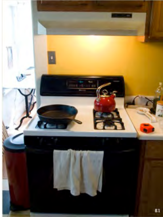
Figure 39. Exhaust System B1; note hallway at left.
