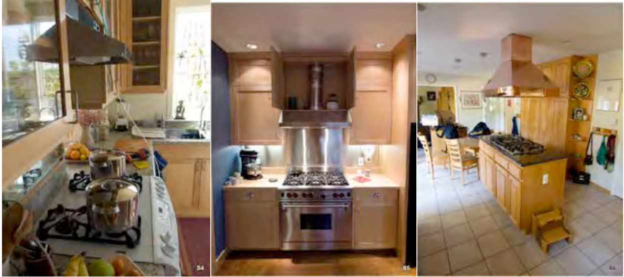
Figure 7. Exhaust systems with open capture hoods B4–B6
