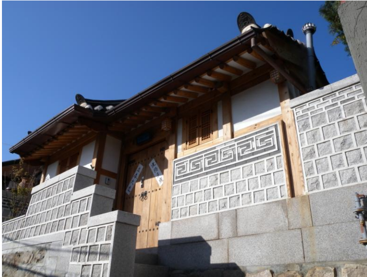
Figure 2.3. Most of the remodeled hanoks in Bukchon, like the one shown in the photo, are wooden post-and-beam structures.
