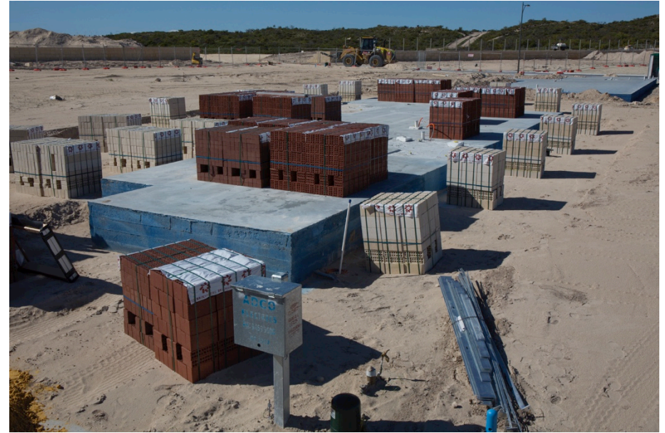
Figure 10. Case 4 (Escarpment): view of dwelling with thickened slab to accommodate site grades (Author 2015).
