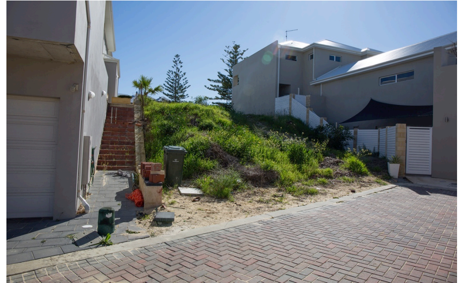
Figure 9. Case 3 (Harbourside Village): view of vacant split-level lot with developed split-level dwellings on either side (Author 2015).
