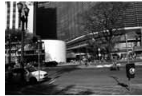
18. Copan, view of entrance hub on Avenida Ipiranga, 2009.
