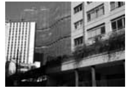
30. View of Copan and neighboring buildings seen from a nearby street, 2009.
