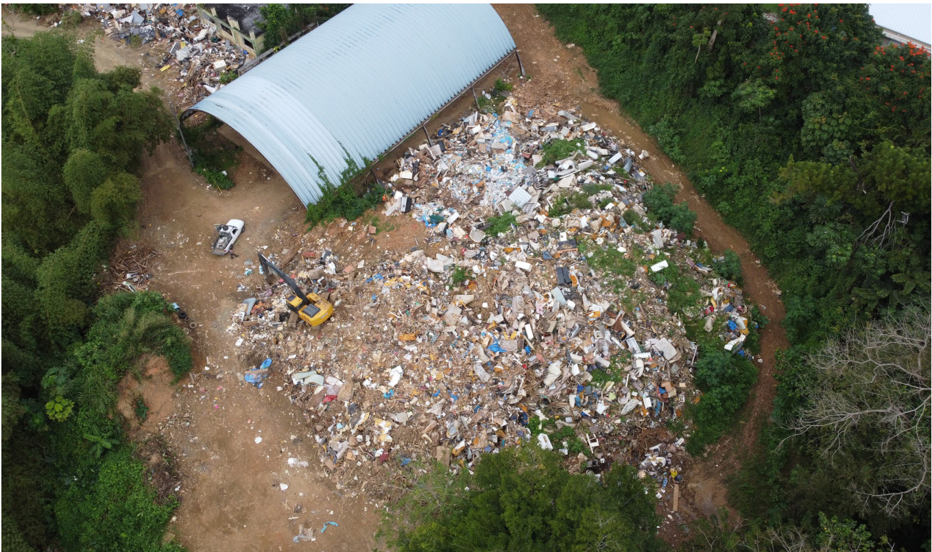
FROM TOP The Josefa Pastrana school in Aguas Buenas has been stripped of doors, windows, air conditioning units, copper wiring, and plumbing.
