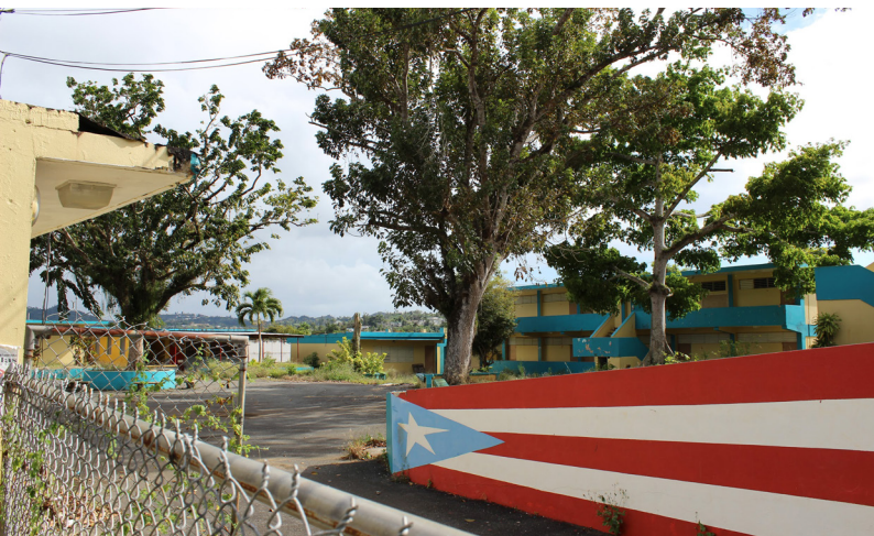
LEFT The Luis T. Baliñas school in Aguas Buenas, shortly after its closing.
