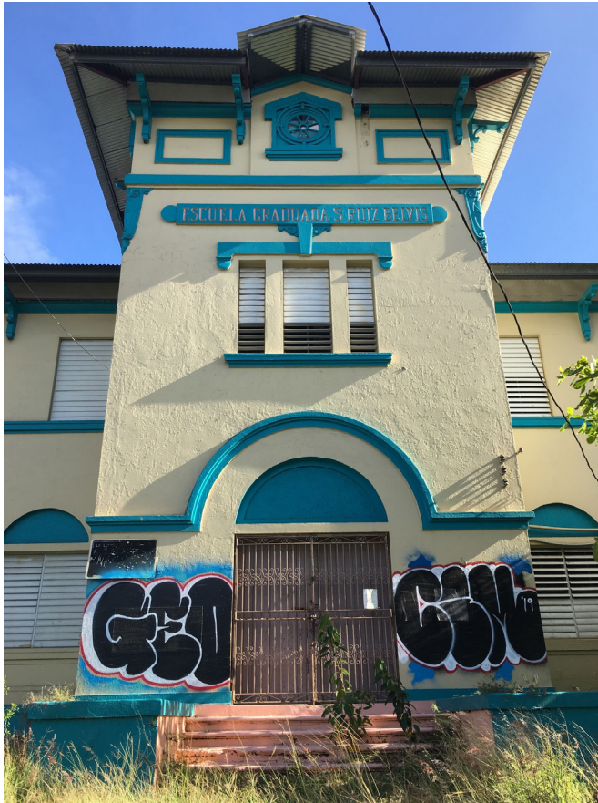
Segundo Ruiz Belvis school in San Juan. The building has both architectural and historic value as a memorial place for its namesake, who was a Puerto Rican lawyer, philosopher, abolitionist, and pro-independence advocate. The marble slab covered by graffiti describes Belvis.
