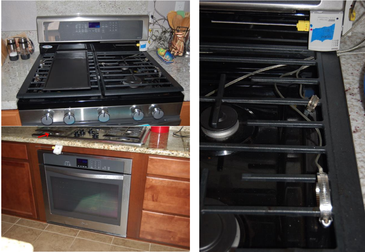
Figure 1 Wire braid thermocouple (five total: left-front, left-back, right-front, right-back, and center of the burner top) and thermocouple probe used to measure cooktop and oven use in House 1 (top left and right). The red arrow shows where one of the four iButton temperature sensors were placed near the left-front burner top in House 2 (bottom left).
