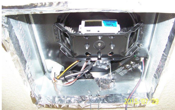
Figure 2 Digital anemometer (upper) and motor state logger (lower) used to monitor bathroom exhaust fan use.
