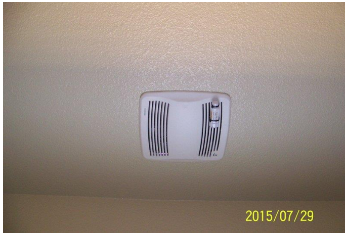
Figure 16 Data logger measuring temperature and relative humidity that was attached to a bathroom exhaust fan grille.
