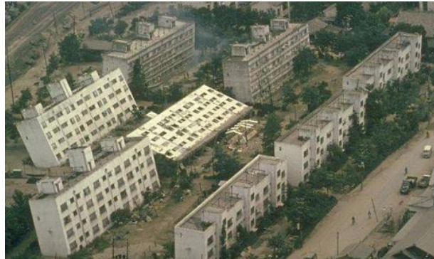
Figure 2.1: Soil Liquefaction, Niigata 1964 ( Japan National Committee on Earthquake Engineering, 1964 )
