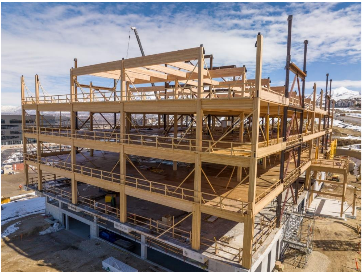
Figure 1 – Multi-story MT structure under construction in Utah, United States
