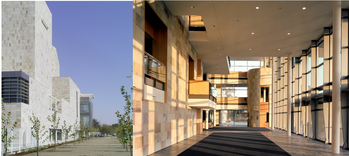
Figure 3.5.1 Outside sandstone wall (left). Figure 3.5.2 Yocha Dehe Grand Lobby sandstone wall (right). Photographs source: Regents of the University of California.
