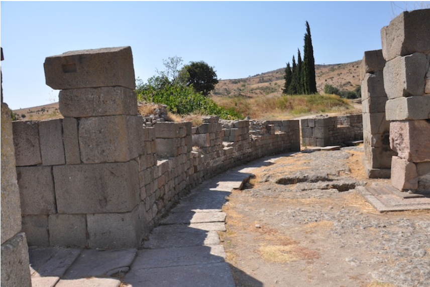
Figure 44 View from ground floor of LRB showing openings towards SW, photo by the author
