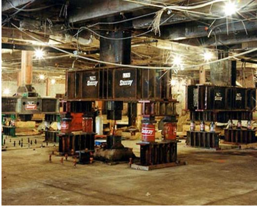
(a) Implementing base isolation
