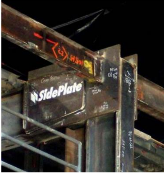
Figure 2.7 Upgrade of Pre-Northridge beam-to-column connections using side plates (photo courtesy of SidePlate System, Inc.)
