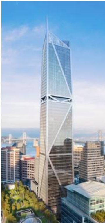
Figure 4.45 181 Fremont at San Francisco (photo courtesy of Arup)
