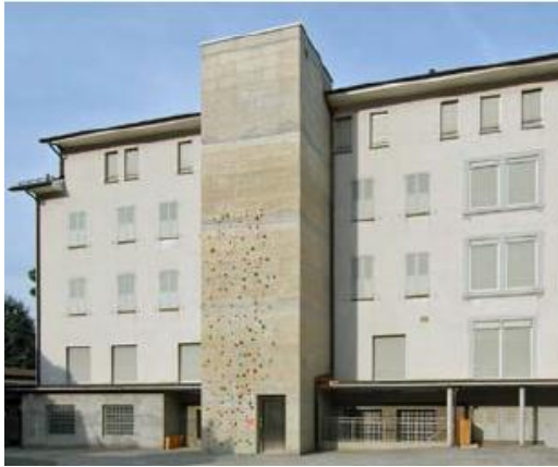
(a) Rear façade after retrofit
