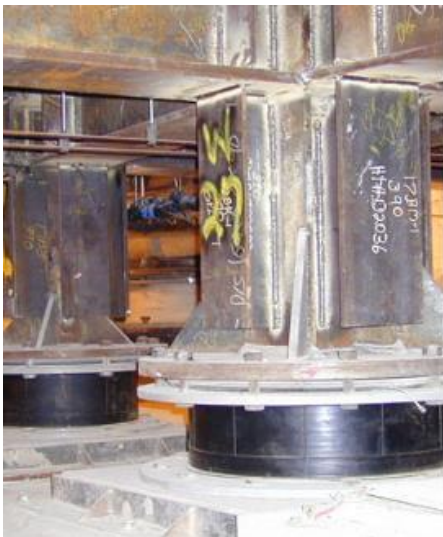
(a) Flat sliding bearings
