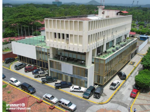
(a) Remaining government offices after removing damaged upper floors
