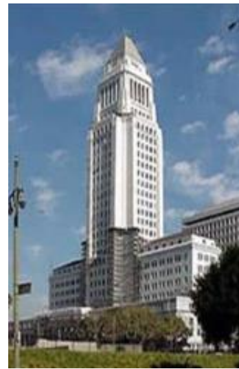
(b) 23-story Los Angeles City Hall
