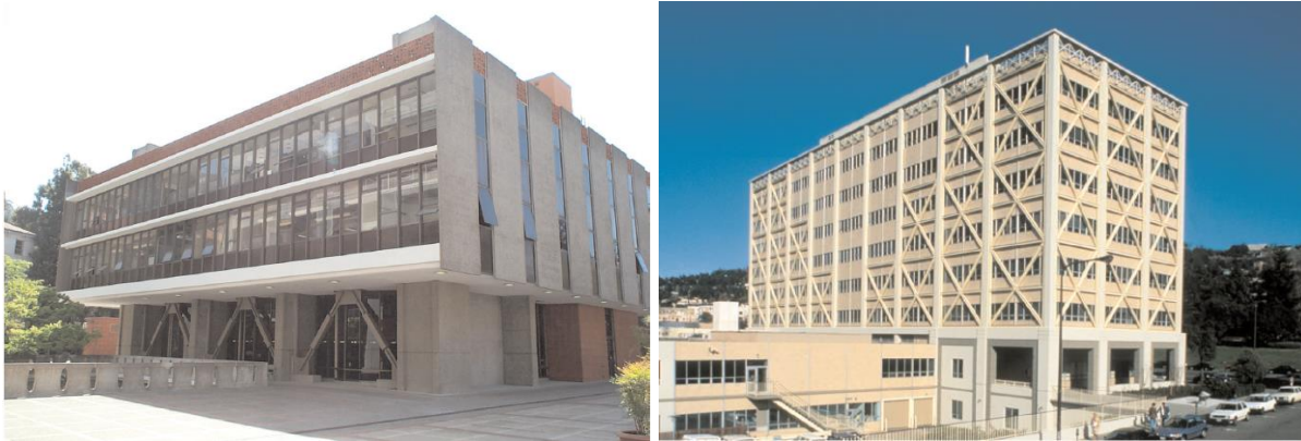
(a) Retrofit of Hildebrand Hall at UC Berkeley (b) Retrofit of University Hall of UC Berkeley
