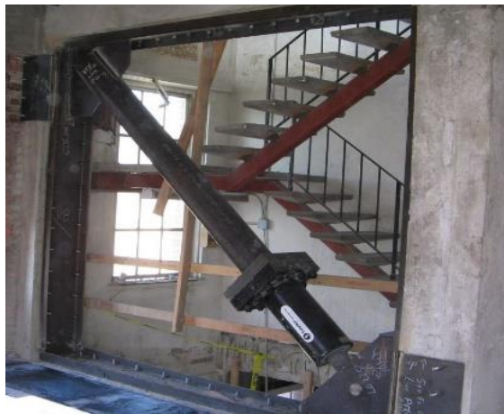
(a) Fluid viscous dampers (photo courtesy of Taylor Device, Inc.)
