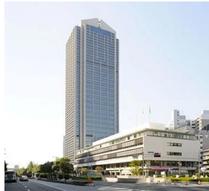
(a) Removal top 3 floors after earthquake
