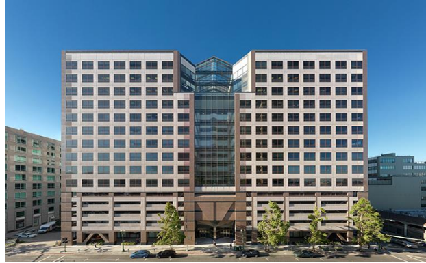
Figure 2.6 Caltrans District 4 office building after retrofit (photo courtesy of Degenkolb Engineers, Inc.)
