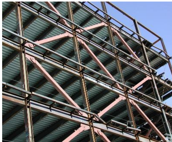
(b) Buckling restrained braces (photo courtesy of CoreBrace, LLC)
