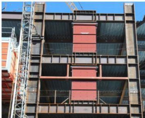
(c) Viscous wall dampers (photo courtesy of Dynamic Isolation Systems, Inc.)
