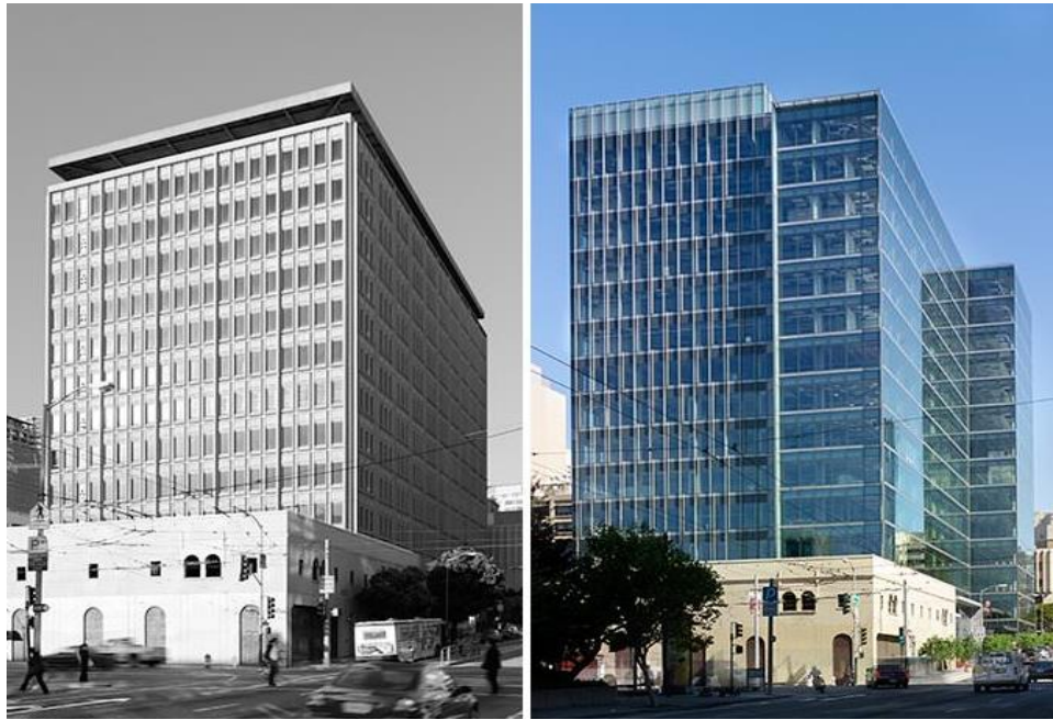
(a) Original concrete façade
