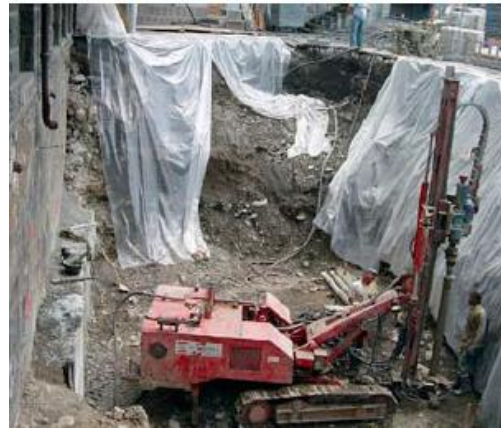
(b) Construction of foundation with micro-piles
