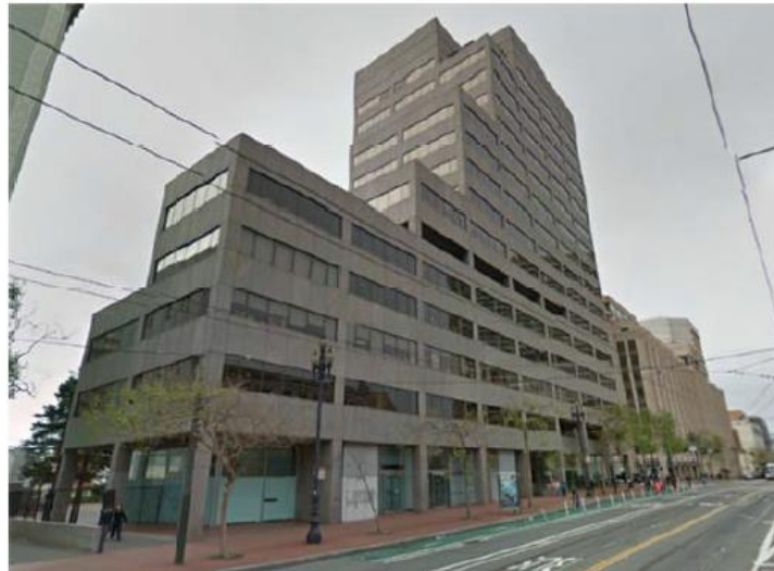
(a) Building after retrofit
