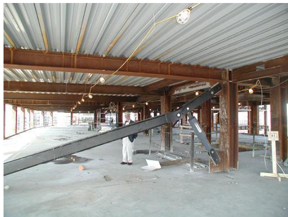
(c) Toggle-brace-damper system
