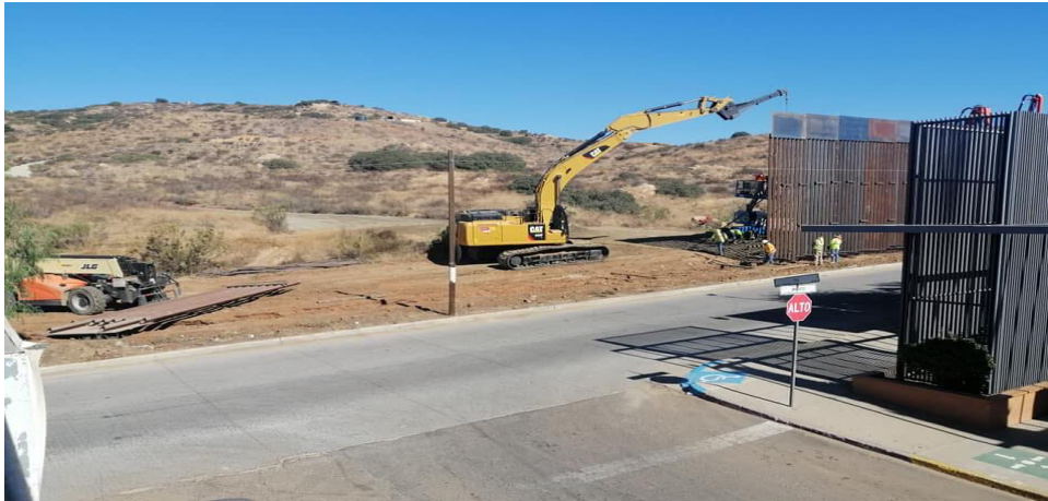
Figure 11 Image taken from Tecate Baja California showing how the U.S. started construction on the wall. The heavy machinery is removing the rusty border wall. We get a glimpse of the border left exposed making visible Campo Indian Reservation.
