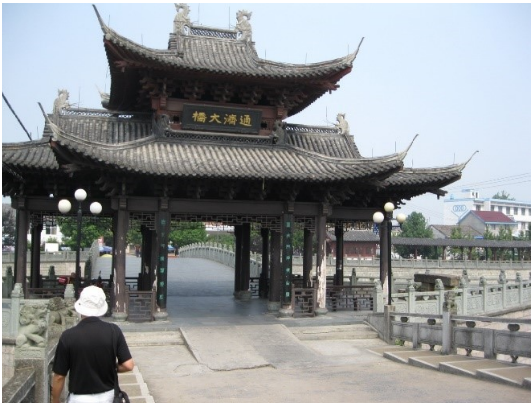
Fig 31 – Yong Village 02, canal bridge and heritage building, public domain
