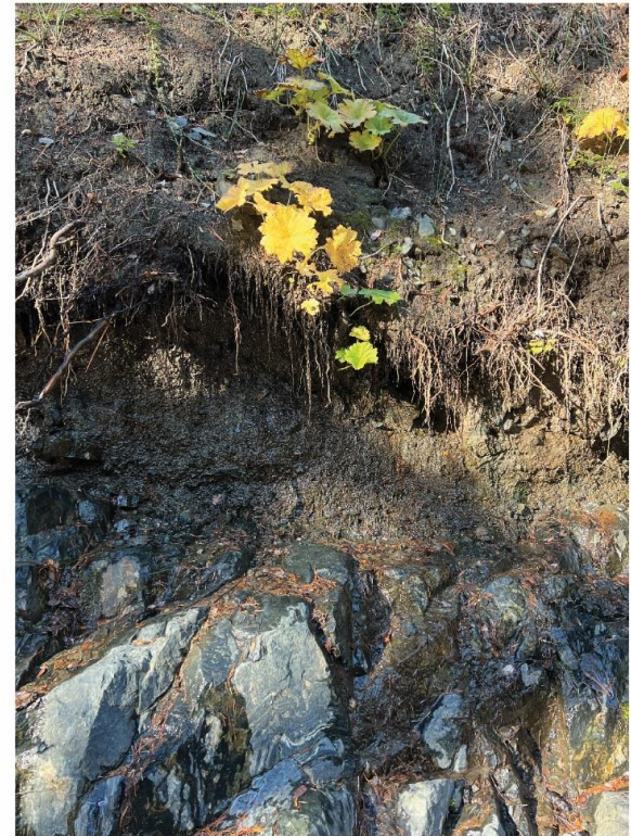
Figure 7d. Evidence of scour on the left bank (looking downstream) from exposed roots.
