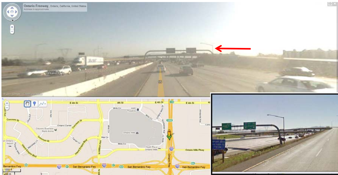
Figure 3-51: Ontario Freeway, next to the 108/109 exit sign at Lat/Lng 34.071191, -117.545297
