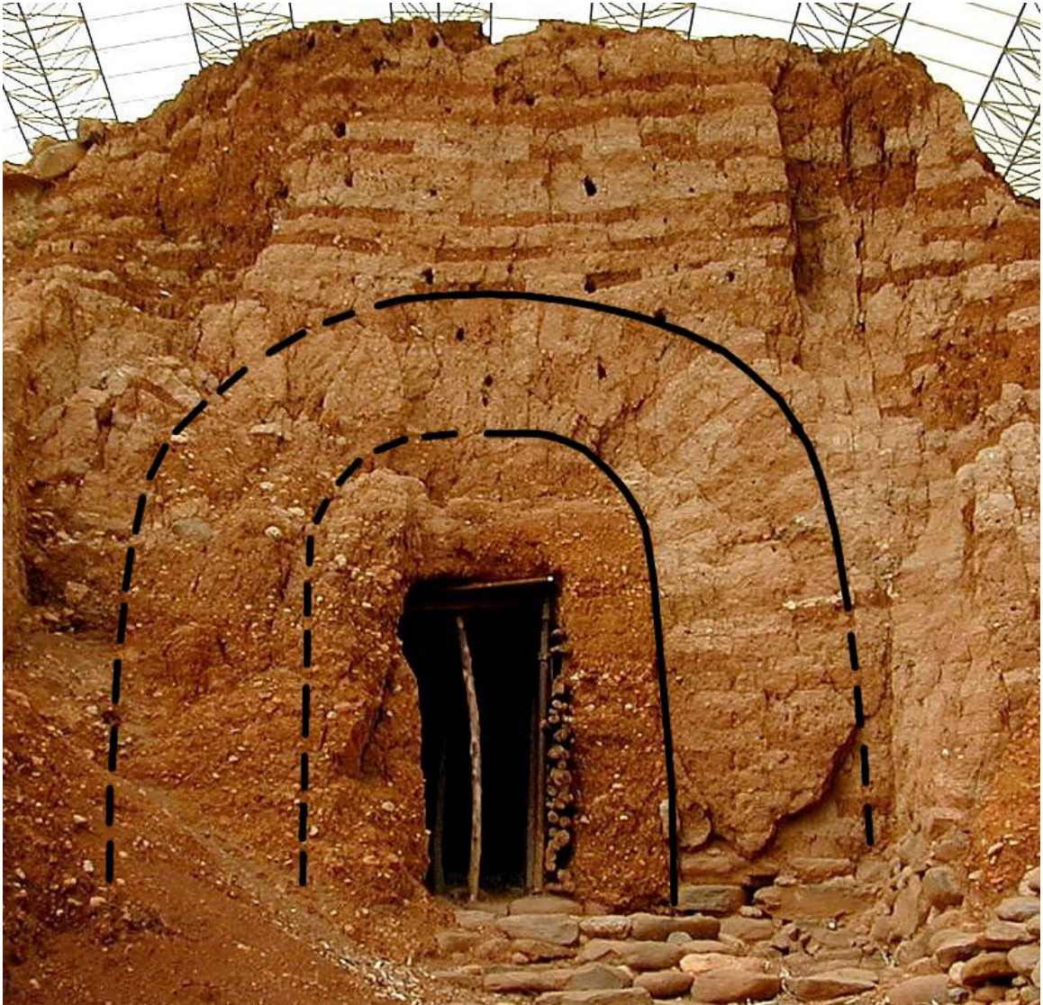
Figure 3.12. The mudbrick arch (traced in the photo) on the façade of Tel Dan’s MB gate, which spans the outermost set of piers. 1 (Note that the original entrance has been only partially cleared.)
