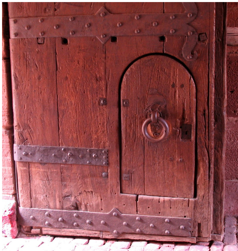
Figure 4.5. A small wicket door built into a gate leaf (here, in a medieval castle) for pedestrian traffic. Heidelberg Castle, Germany. 1
