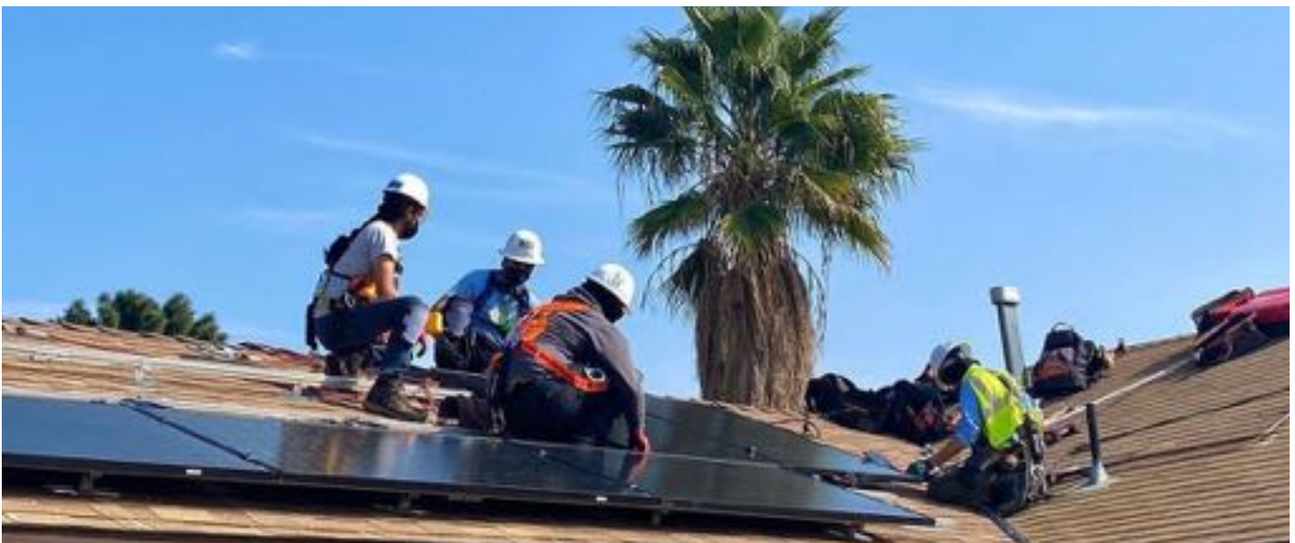
GRID Alternatives Solar Installation on a resident's home in Pacoima on March 2022 . Source: GRID Alternatives GLA
