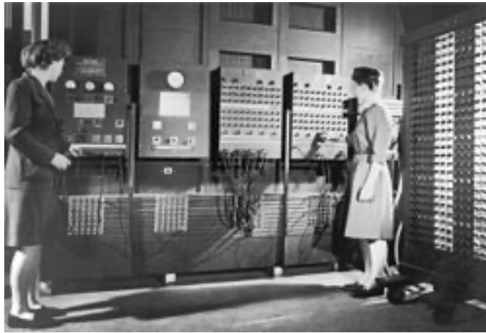
Figure 1.3 Programmers operate ENIAC's main control panel at the Moor School of Electrical Engineering. This picture is in the public domain in the US and taken by United States Army
