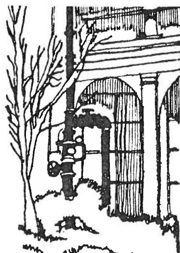
An indication of change: outside utility plumbing added to original home.
