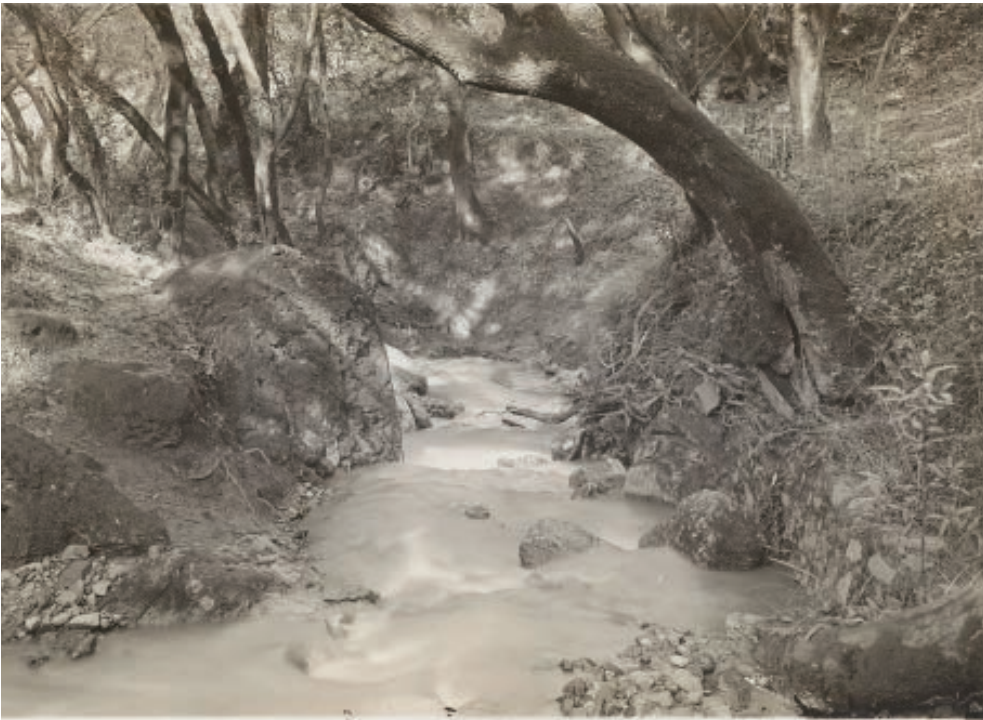
Fig. 1 Strawberry Creek's original flow photography by L.S. Smith Feb 1916.
