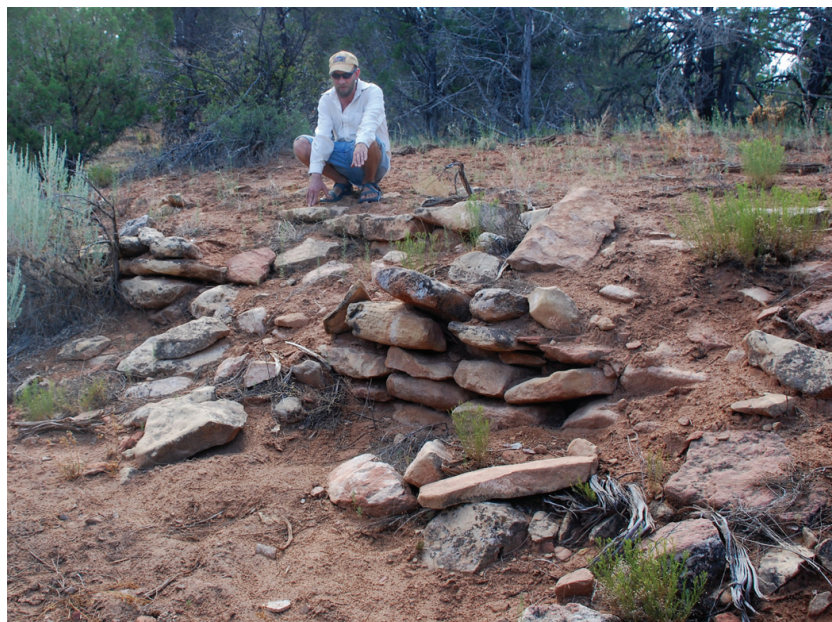
Figure 3.9. Photograph of the retaining wall at the Red Knobs Annex.
